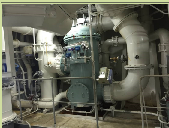
Ballast water treatment system. Photo provided by, Marc Gagnon, Fednav.
